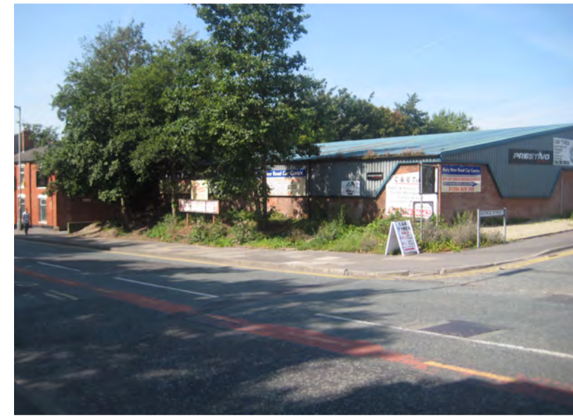
Britannia Mill Industrial Estate - Remove redundant signage, construct low brick retaining wall, remove weeds and apply a low maintenance treatment to the bank
